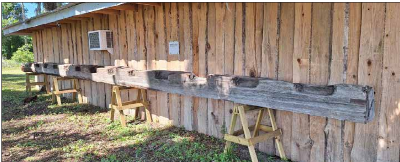
This 40 foot long post was hand-hewn from a live oak tree and is the original beam from the local grits mill, Allen Mill/Pond Grits Mill. Locals would bring large sacks of corn by mule to grind down into grits for their families.
